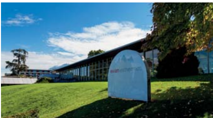
The spa was designed by French architect Olivier Chabaud and is themed around water
