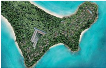
The resort has been designed by Italian architect Paola Navone
